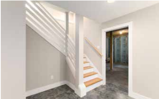
4th Bedroom Ready for Finishing
